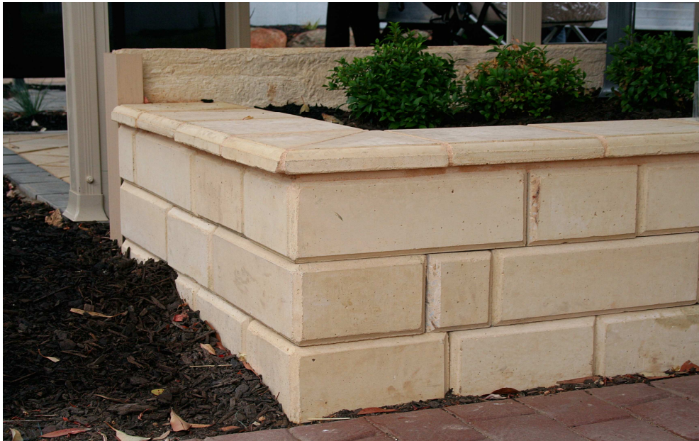
Kimberley Wall - sandstone
